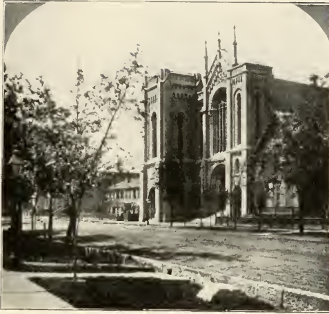
THE FIRST PRESBYTERIAN CHURCH, 1859— WABASH AVENUE, NEAR CONGRESS STREET.
